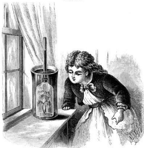
Apparatus arranged to catch the O evolved from a sprig of leaves.
